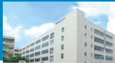
R&D Center in Guangzhou
